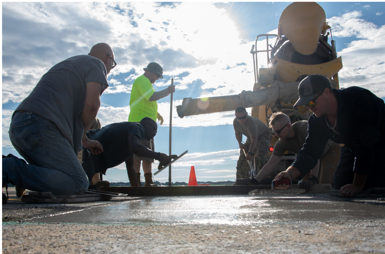
Members with the 316th Civil Engineer Squadron Heavy Equipment Section, known as the “Dirt Boys,” finish smoothing over concrete for repairs on the flightline at Joint Base Andrews, Maryland, Aug. 8, 2023. These repairs help the base save on potential environmental damage costs in the future.
