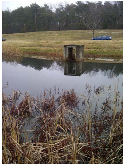
View of: Outlet Structure Facing North
