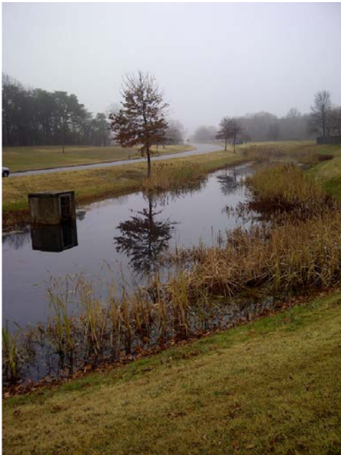
View of: Retention Pond Facing East
